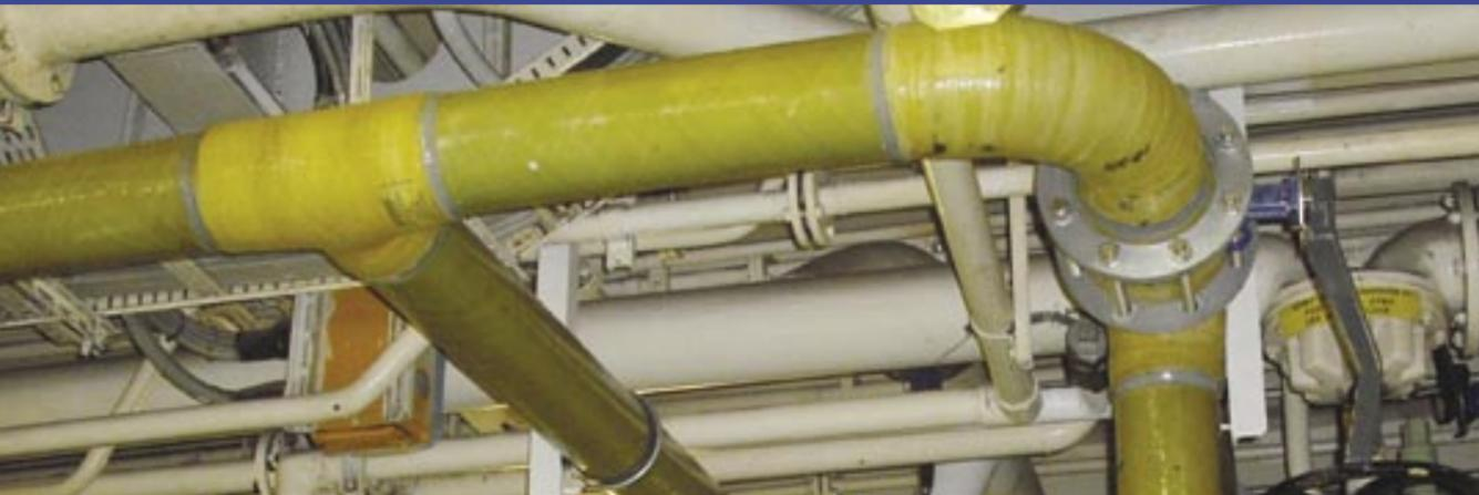
FPI's GRE Wavistrong and Fibermar pipe systems are the ideal replacement for legacy steel systems – GRE's non corrosive characteristics and light weight ensure this. It is simply just "Fit & Forget".
